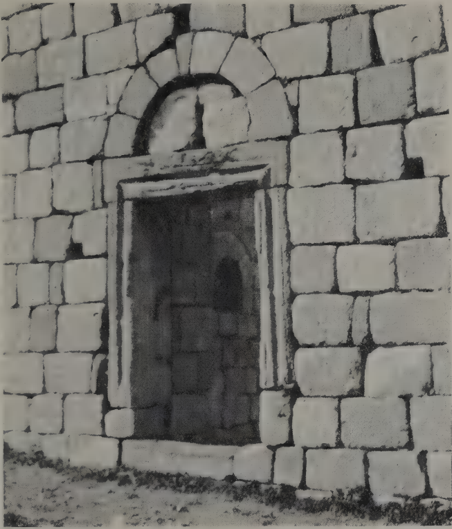
FIG. 169.—No. 43, door in monastery.
